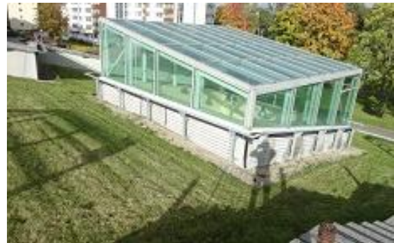
Figure 6. Green roof of shopping centre Olympia (Source: photo by the authors, 2012)
