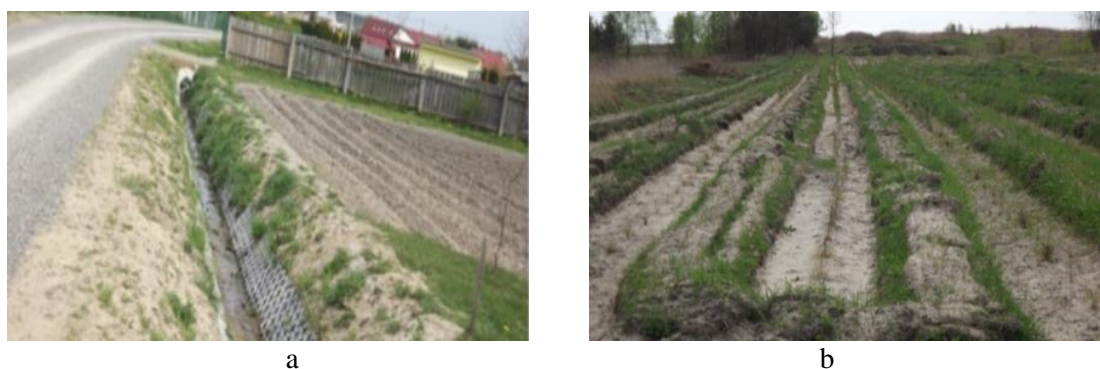
Fig. 1. Implementation of environmental measures during the land consolidation in Hucisko surroundings (Poland): a) – renovated reclamation system and designed culverts; d) the afforestation of unproductive lands (Leń et al., 2016)
